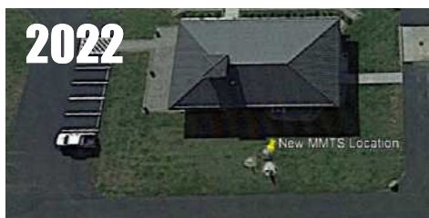
Same location at city WWTP, but MMTS moved to a better location over grass in front of office. Better site, but still too close to road and the building. See markers. RATING = CRN4
