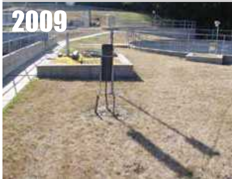
Winnepago, MN , at city WWTP, nearby sewage tanks, concrete pad. RATING = CRN4
