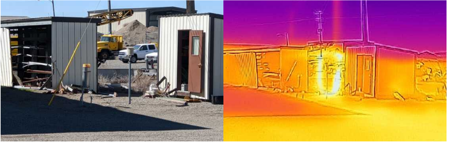
Visible and infrared photos of MMTS placement of GHCN station for Shoshone, ID, next to a junk yard at the city maintenance facility. The station is surrounded by heat sinks. Source: Anthony Watts.
