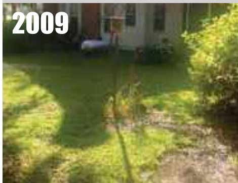
Union Springs, AL , nearby building. RATING = CRN4
