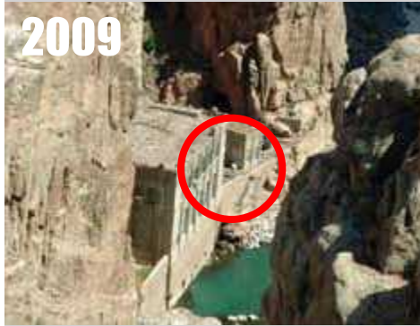
Buffalo Bill Dam, WY , sited on concrete, between two buildings. RATING = CRN5
