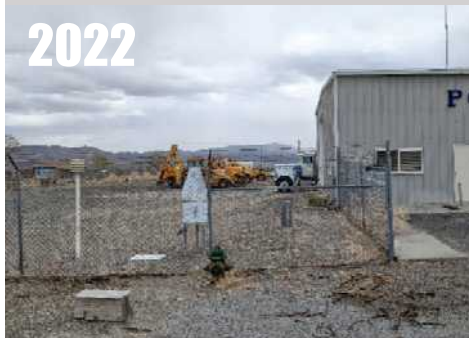
Closed, then moved to an industrial area, worse location. RATING = CRN5
