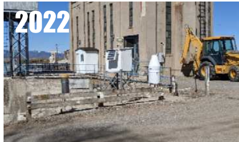
No change to location, but MMTS added improperly to the roof of the CRS, resulting in warmer temperature. RATING = CRN5
