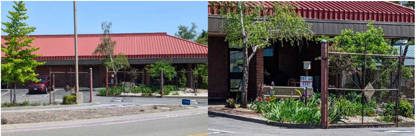
MMTS placement at the Auburn, CA, post office, a GHCN station. Note the multiple heat sinks near the sensor, which is surrounded by asphalt, concrete, and brick buildings. Source: Anthony Watts.
