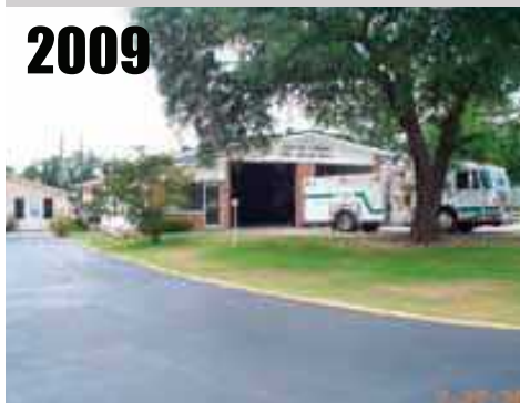
Conway, SC , near large asphalt area, building. RATING = CRN4
