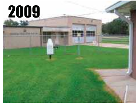
Bunkie, La , too close to sidewalk and Building at WWTP. RATING = CRN4
