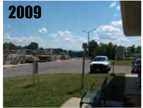
Lexington, VA, sewage plant, near building, sidewalks, road, parking lot at WWTP. RATING = CRN4
