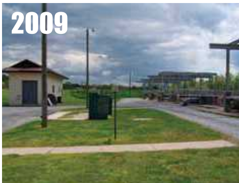
Tullahoma, TN , at city WWTP, electrical transformer, cement path. RATING = CRN5
