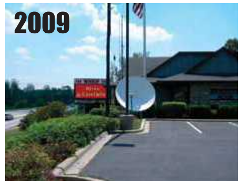
Hendersonville, NC , nearby parking lot, satellite dish, building. RATING = CRN5
