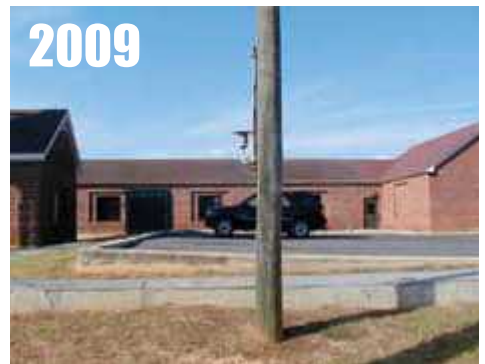
Orangeburg, SC , nearby metal coverings, parking lot, building at WWTP. RATING = CRN4
