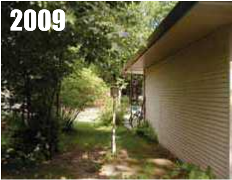
Crosby, N.D. , nearby building, patio. RATING = CRN4
