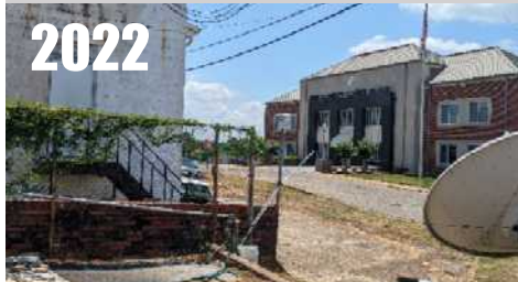
Same location, but MMTS was moved to top of brick wall, closer to building and parking lot. Worse siting than original. NWS seems unaware of move, no mention in HOMR. RATING = CRN5
