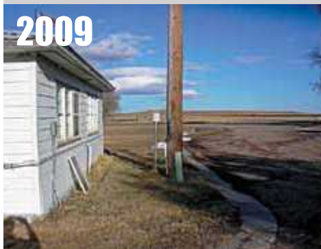
Hay Springs, NE , next to building, narrow sidewalk, telephone pole. RATING = CRN4
