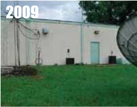
Greenville, TX , nearby building, satellite dish, two air-conditioning units. RATING = CRN4
