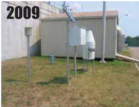
Staunton, VA , at WWTP, between tank wall and paved road. RATING = CRN4
