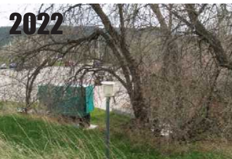
MMTS remains partially obscured by foliage, but new generator has been installed nearby. RATING = CRN3
