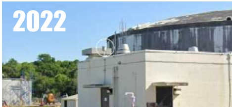
Same location at WWTP, but NWS reports: "MMTS MOVED 102 FEET SOUTHEAST." However, new site on rooftop is just as bad if not worse than original siting. Note exhaust fan nearby. RATING = CRN5
