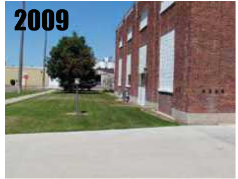
Rock Rapids, IA , nearby building, sidewalk, driveway. RATING = CRN4
