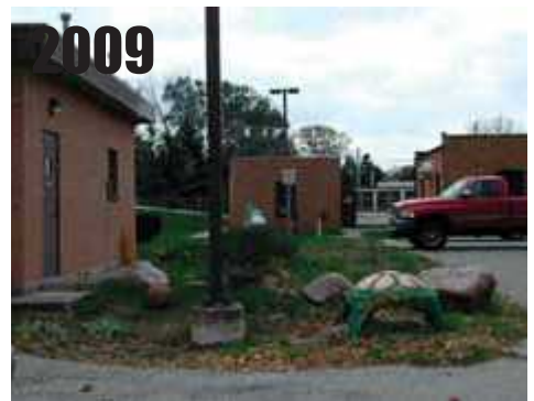
Marengo, IL, nearby buildings, parking lot at WWTP. RATING = CRN4
