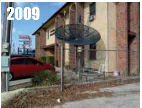
Lampasas, TX , next to sidewalk, near satellite dish, road, parking lot, building. RATING = CRN5
