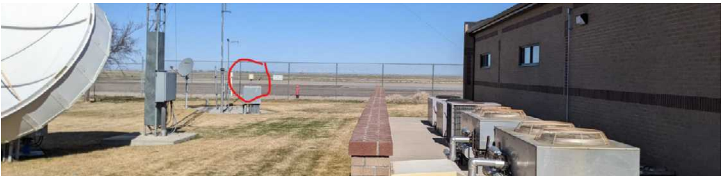
GHCN station at the rear of the Pocatello, ID, National Weather Service Forecast Office. Note the bank of a/c units on the right, the MMTS (circled in red) and the airport tarmac in the background. Source: Anthony Watts.
