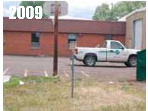
Gunnison, CO , nearby parking lot. RATING = CRN4
