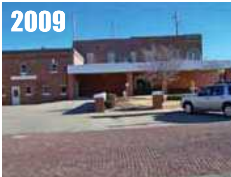
Fort Scott, KS , overwhelmed by large paved area, nearby building (Funeral Home). RATING = CRN5
